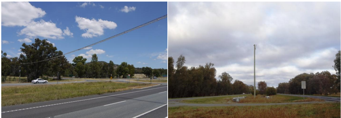
Figure 1. A rope bridge (left) and glider pole (right) installed along the Hume Freeway in north-east Victoria.
